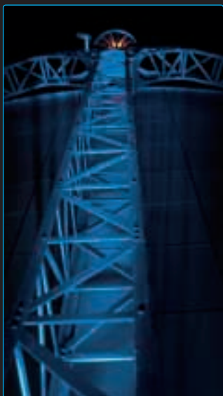
revealing the structure
