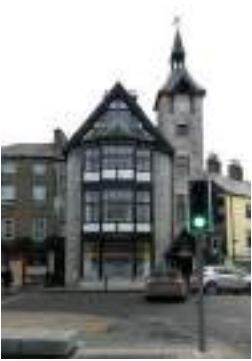
[96] Mallow_35 Bridge Street
